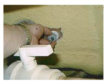
You will simply need to thread the retaining nut on and tighten it down. Insert the temperature sensor into the well assembly, and push the rubber grommet in to lock the sensor in place.
