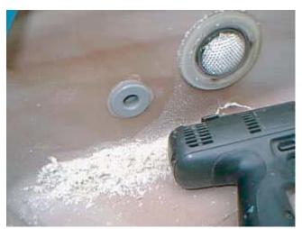
When you are ready to install a thermowell for your new electronic temperature sensor, you usually want to pick a flat spot somewhere easy to get to, approximately halfway below the water level. This will ensure that the temperature reading reflects more of an 'average' temperature of the water. You can use a 1.125" (1 1/8") hole saw bit to make the hole.
