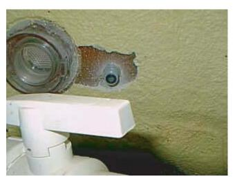
After pushing the thermowell through the shell, the next thing you'll want to do is to apply additional silicone sealant around the back of the thermowell, where it meets the fiberglass shell. IF YOUR THERMOWELL CAME WITH A GASKET, DISCARD IT! Use the silicone sealant to insure a truly watertight seal.
